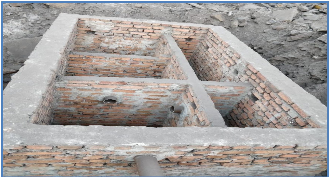
Picture 10 – Oil & Grease Trap
